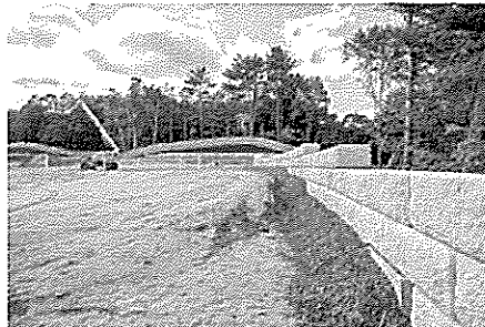
Retaining Wall Completion
