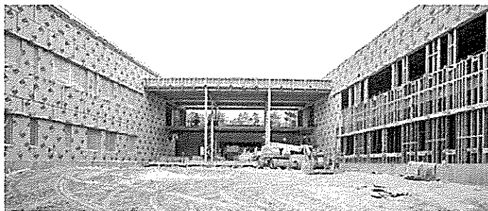
B and C Wing Exterior Wall Progress
